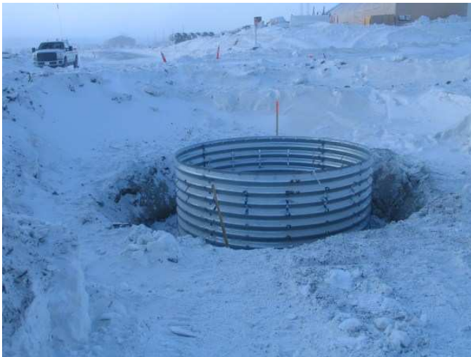
Photo 5: Sump 2 installed.
