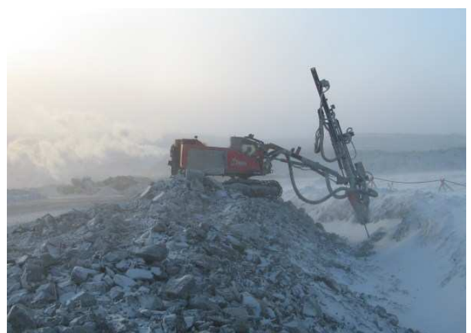
Photo 8: Drilling high spots in berm trench
