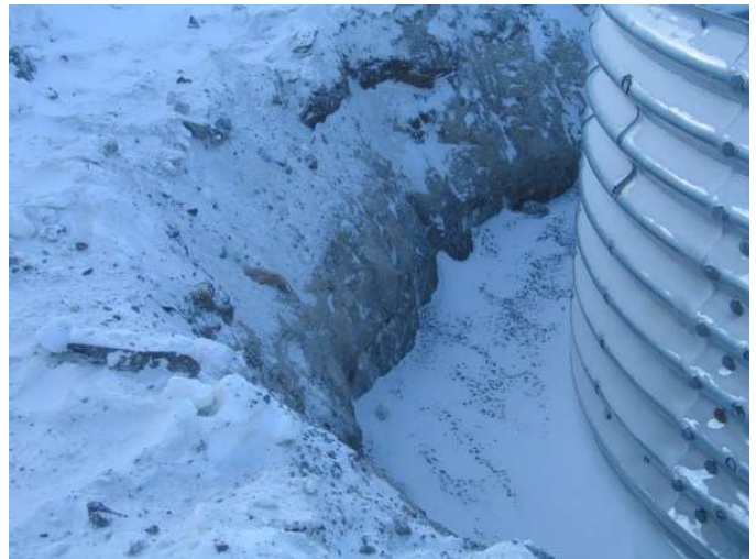
Photo 6: 5/8" crush placed around sump 2.
