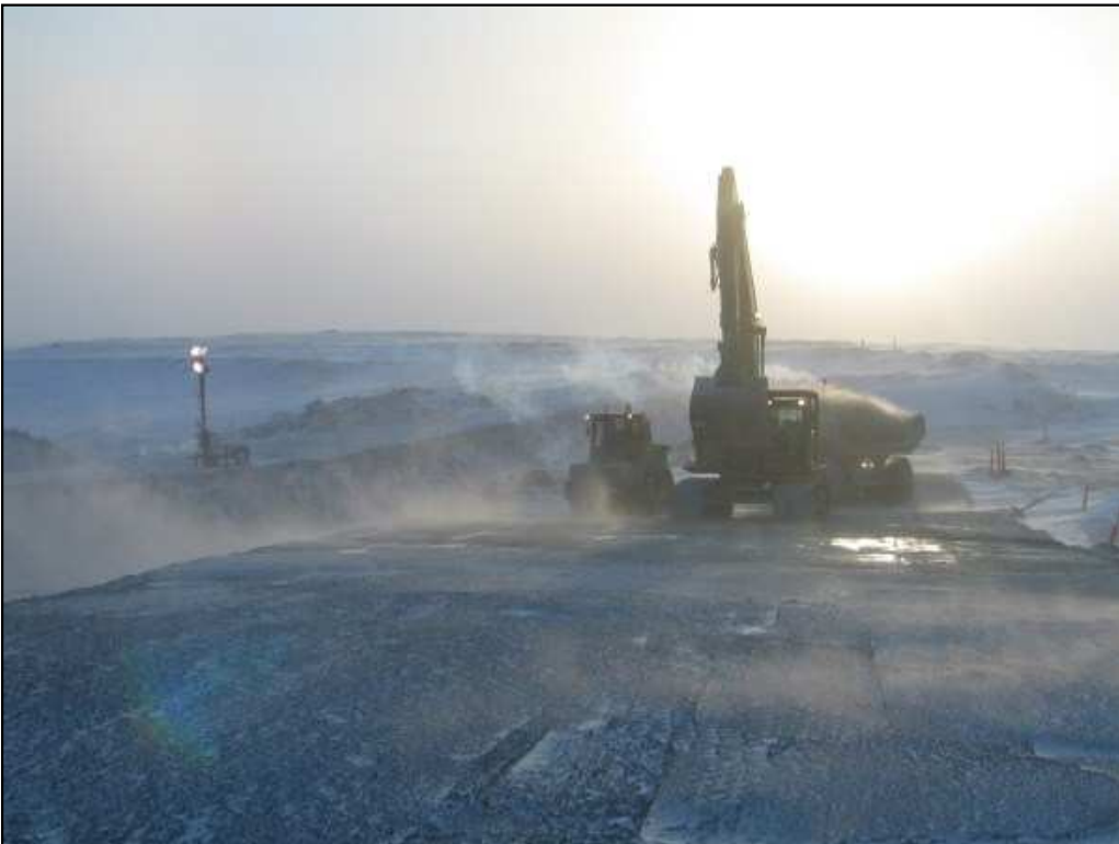
Photo 12: Placing FCM
