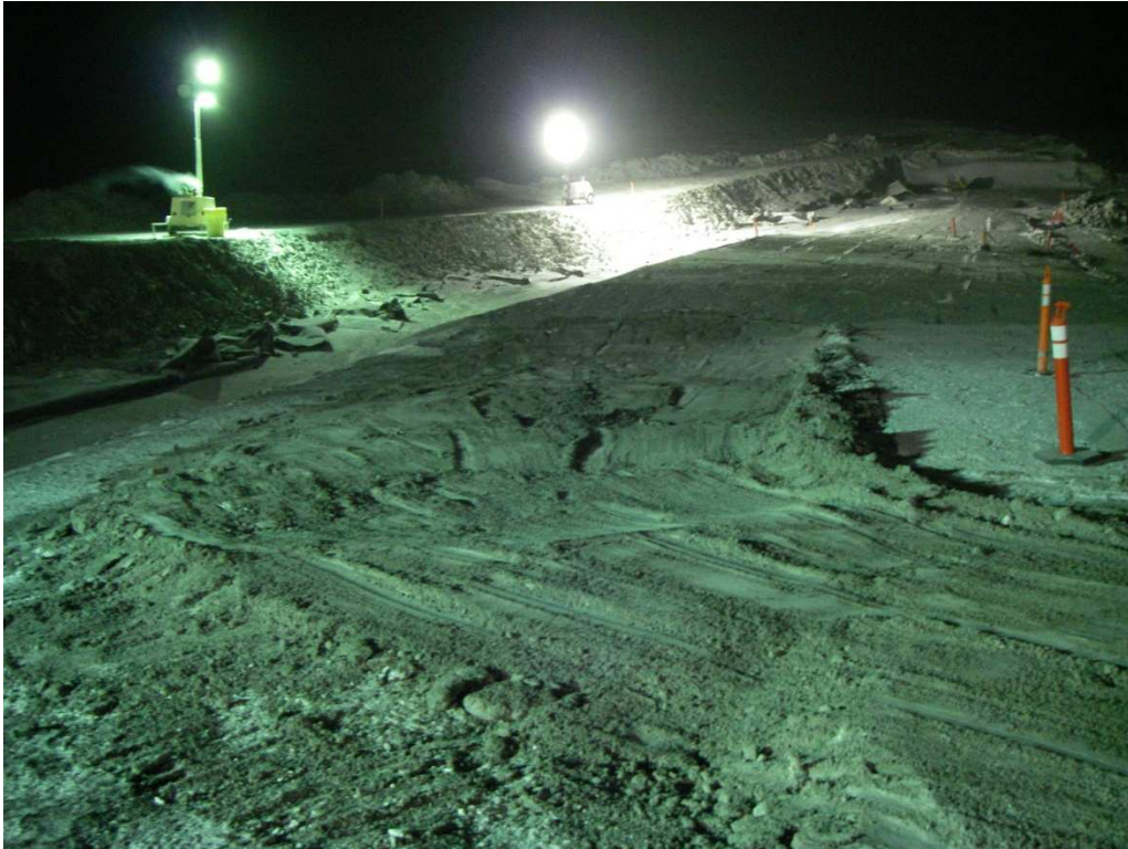
Photo 13: Frozen core area after removal of the sub-standard material.
