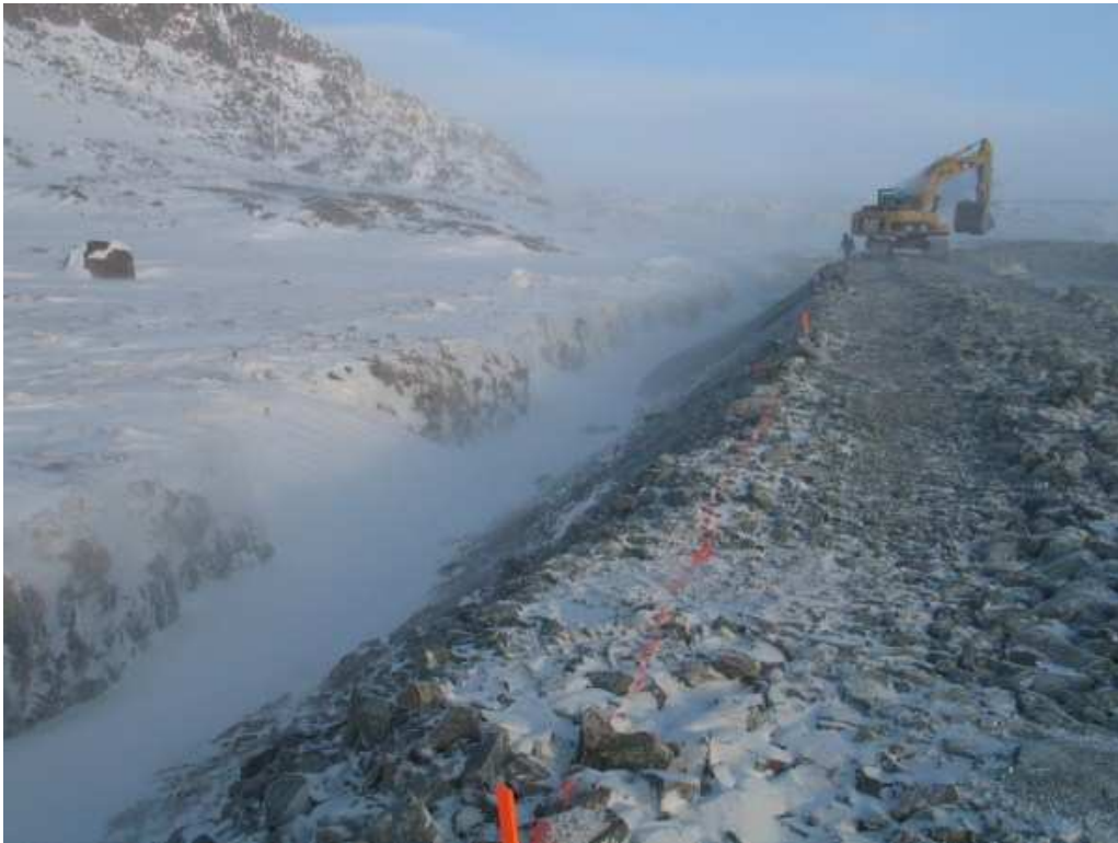
Photo 9: Key at north diversion berm filling with snow.
