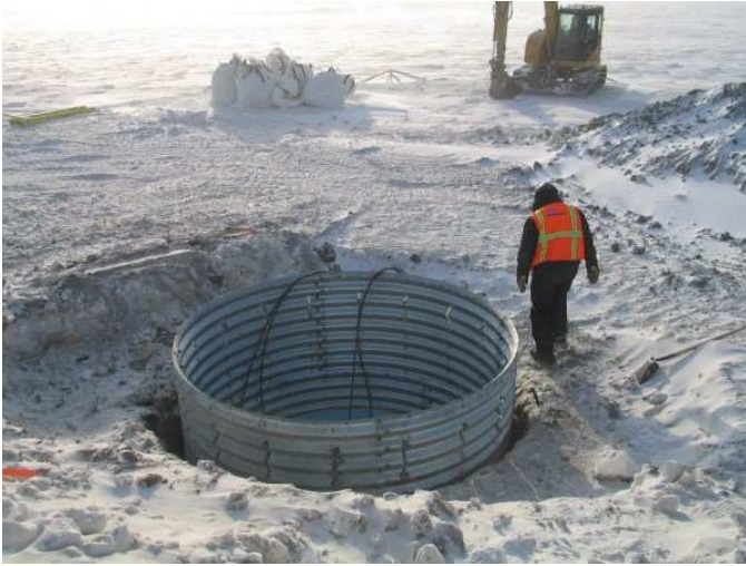
Photo 3: Sump 1 installed.
